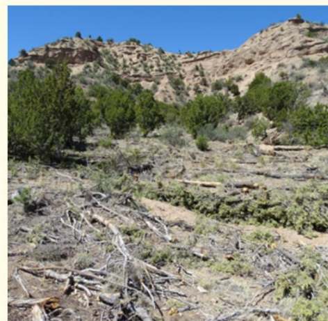
Example how logs on contour, slash on slopes, and wicker weirs together help stabilize sediment and cover bare soil. (photos: Jan-Willem Jansens).
