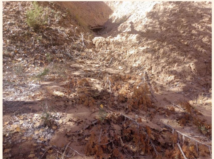
Example of erosion control structures using locally available materials. Lop and scatter of juniper slash slows and spreads flows at the toe of a gully and helps stabilize sediment after peak flows are reduced by a small log rack higher up in the gully's canyon. (Photo: Jan-Willem Jansens)
